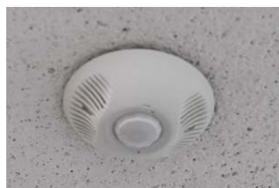
Motion sensors were installed in offices and hallways to reduce energy consumption for lighting at headquarters in 2020.
