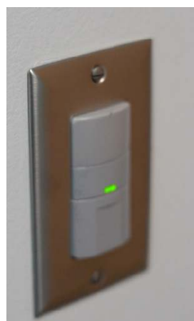
Motion sensors were installed in offices and hallways to reduce energy consumption for lighting at headquarters in 2020.
