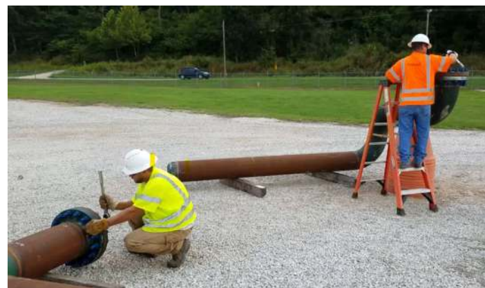
Southern Star team members are preparing sections of pipe for hydrotesting.
