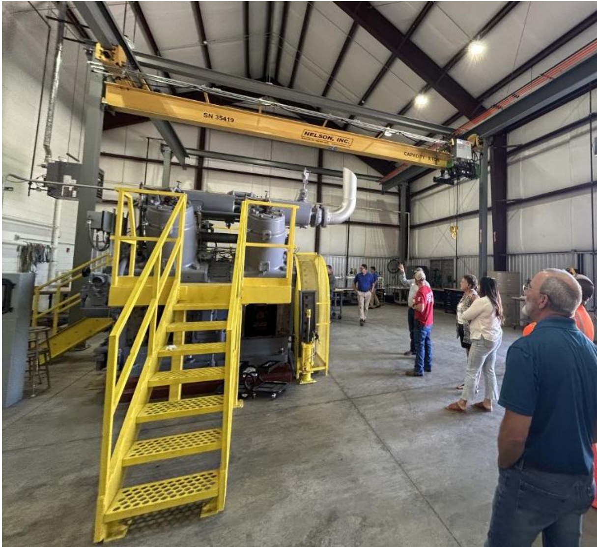
Hesston Training Center hosted a Harvey County (Kansas) Local Emergency Planning Commission meeting on June 20, 2025. These meetings provide an excellent opportunity to connect with local government officials and educate them on pipeline safety and Southern Star’s operations.
